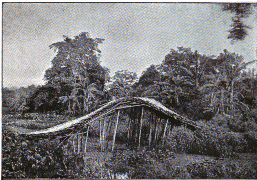
FIG. 1. BRIDGE OVER STREAM AT RANGPUR.
